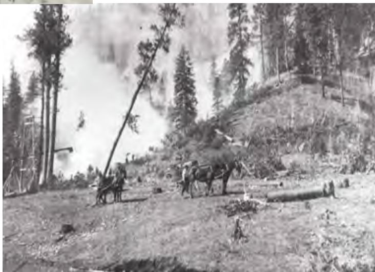
Figure 1.11. Logging on the Pajarito Plateau (Photos on this page courtesy of the Los Alamos Historical Society)
